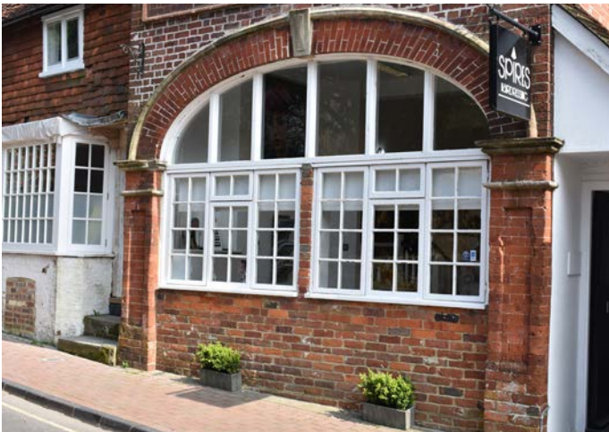
Lunette window at 1 Church Lane
