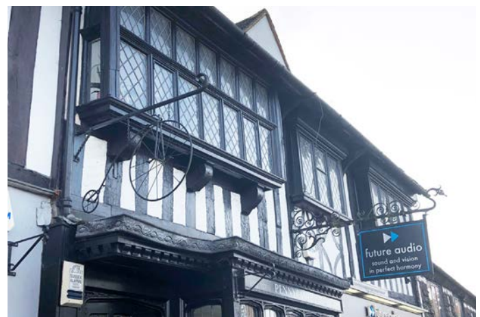
Oriel windows, 30 High Street
