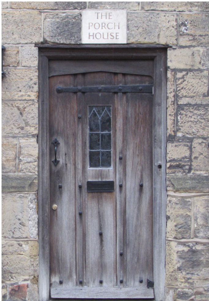
Oak door with iron detail of The Porch House, 82 and 84 High Street
