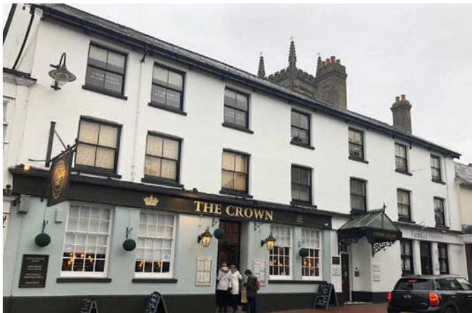
Crown Hotel, 35 and 37 High Street
