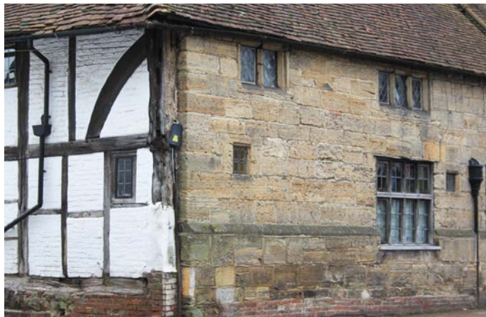
Timber framing and sandstone wall of 84 High Street
