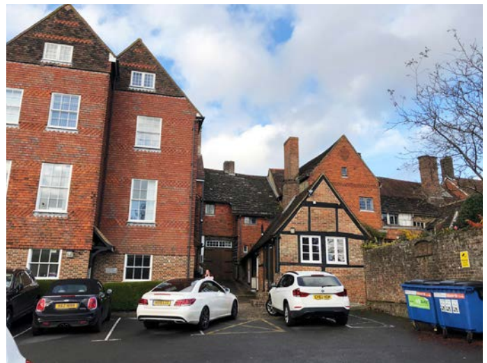
Rear of 58-64 High Street
