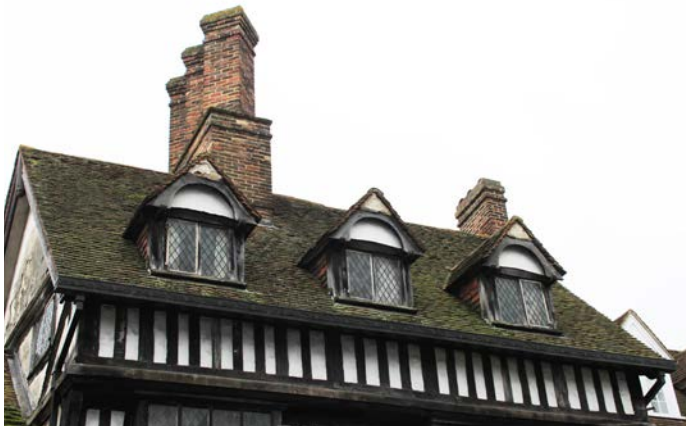
Dormers on Cromwell House, 80 High Street
