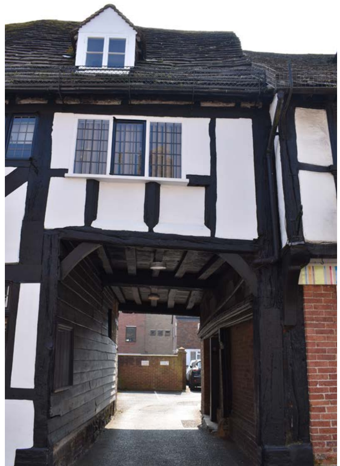
Carriageway between 46 and 48 High Street
