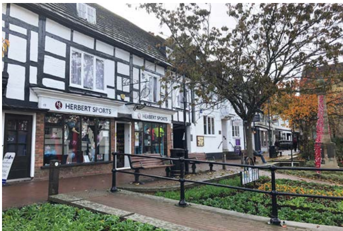
View West along Southern walkway of High Street
