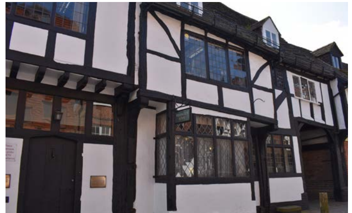
Wilmington House, 48 and 50 High Street
